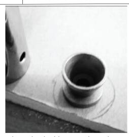
Using the individual bars mark on the wall the position of the required mushroom fixing on the left hand leg side. Attach the mushroom to the wall using the wall plug and wood screw provided.
